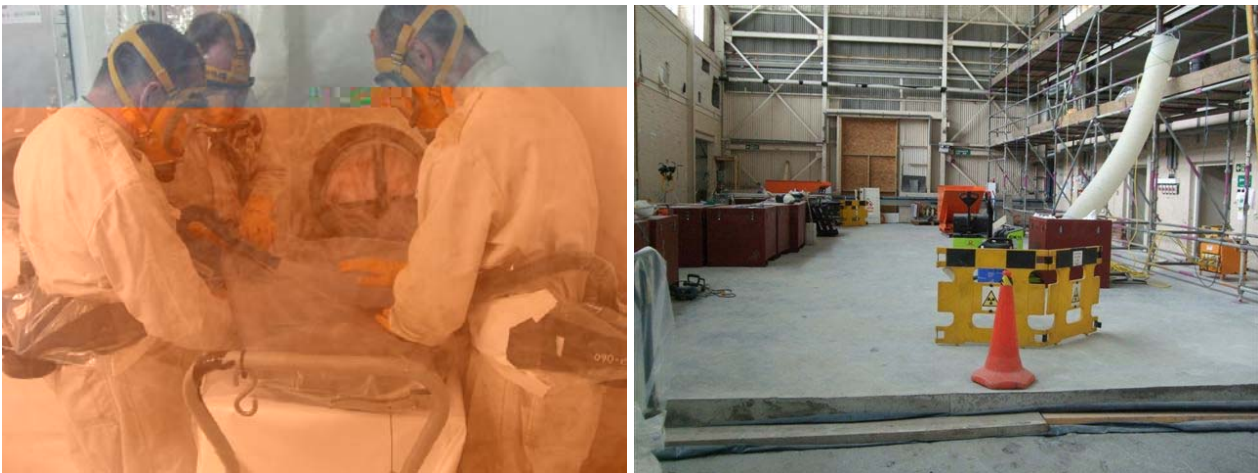
Figures 4 & 5: D1206 Glovebox window replacement preparations and D1207 floor sealing work
