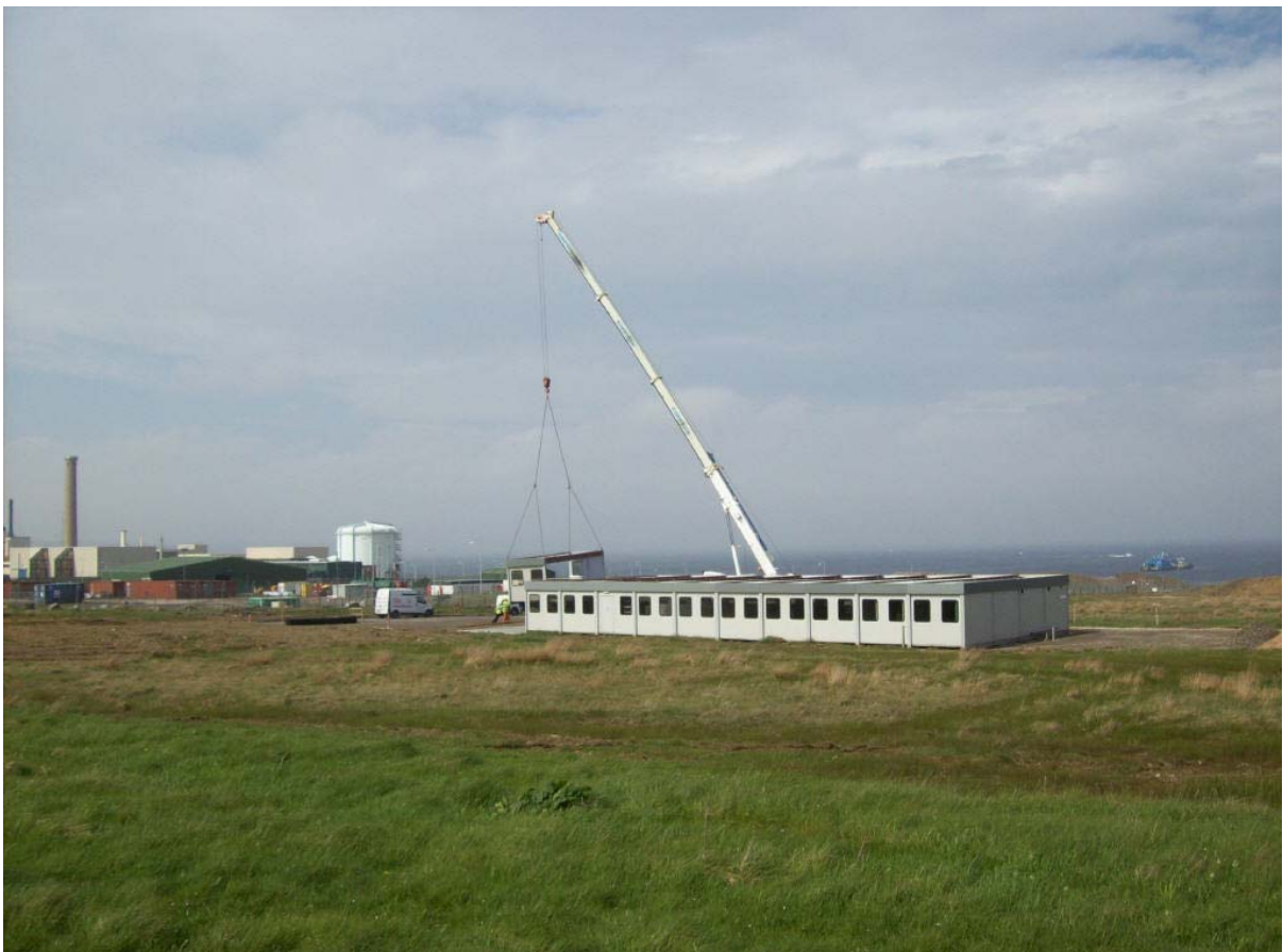
Figure 3: New office accommodation for the D3100 project.
