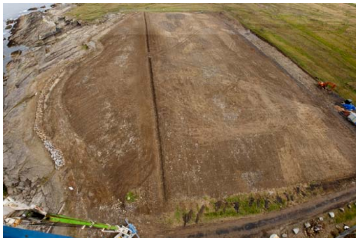
Figures 1 and 2: Aerial views of Landfill 42 after reprofiling
