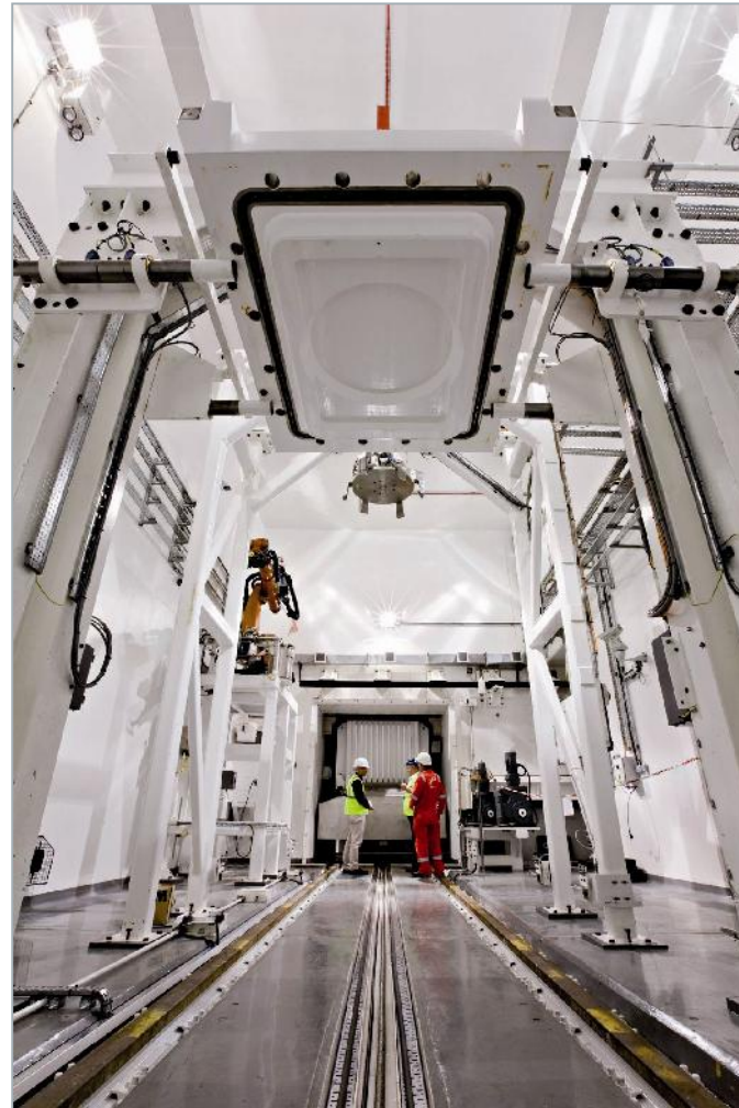
Inside the Breeder Removal Facility at the Dounreay Fast Reactor
