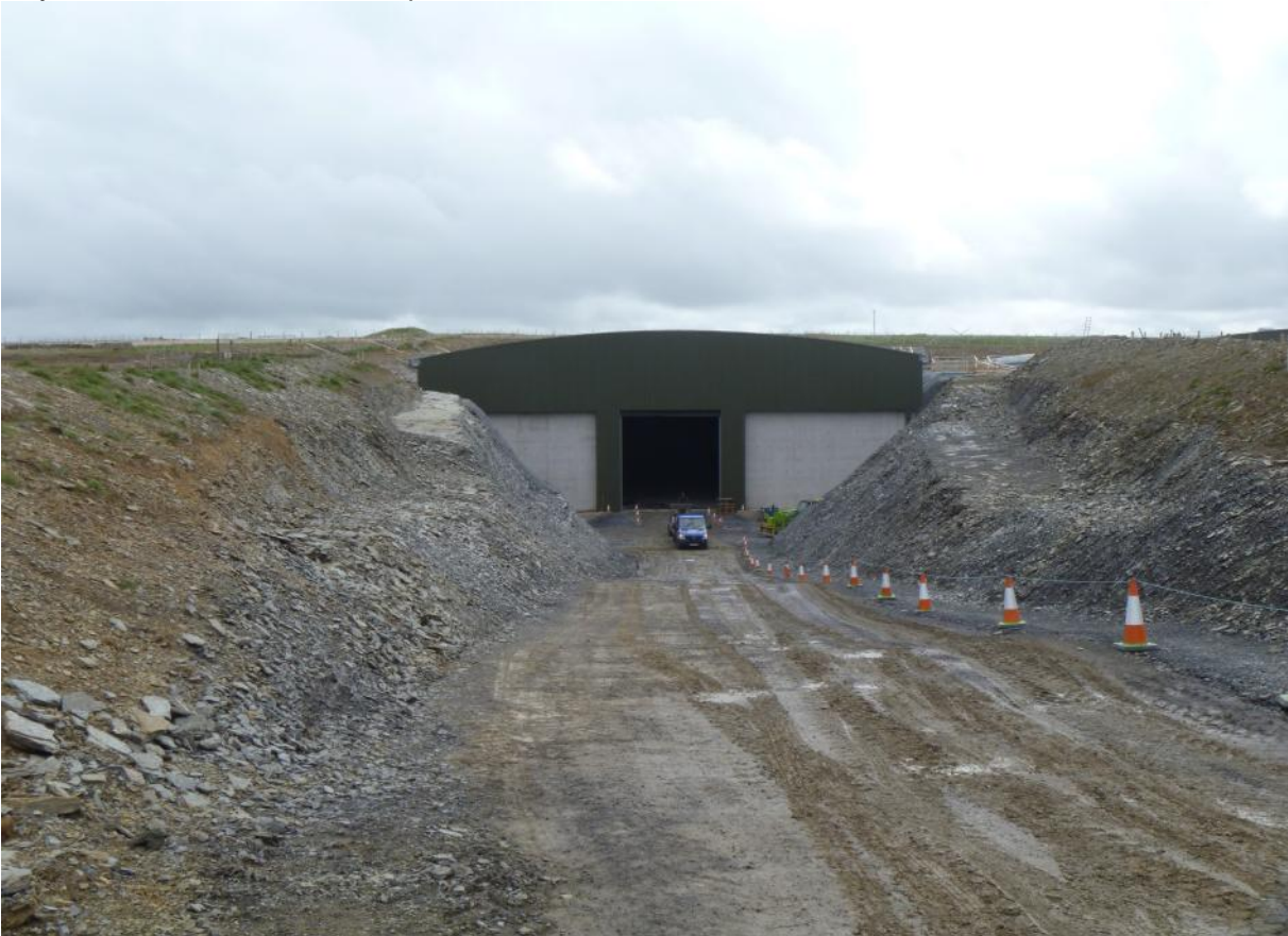
May 2013 – roof installation complete
