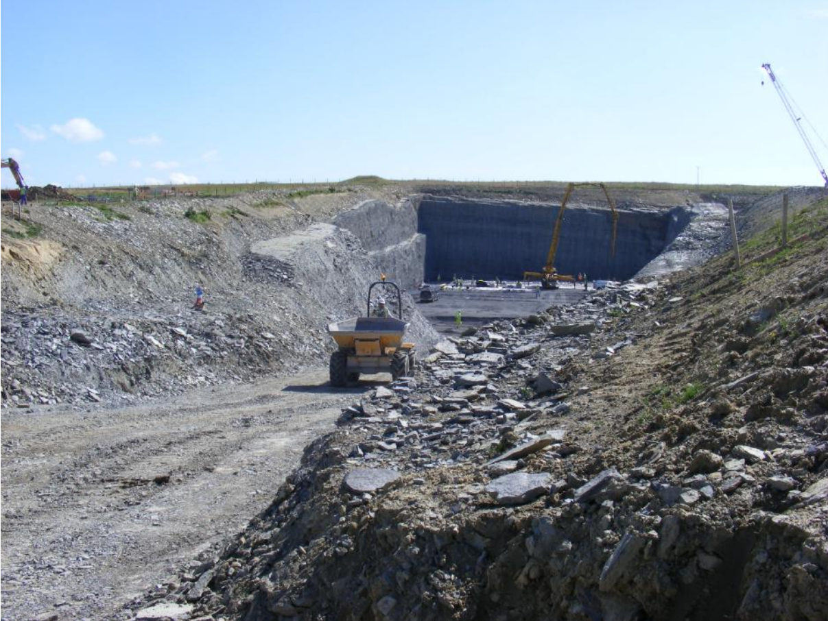
August 2012 – installation of floor slab
