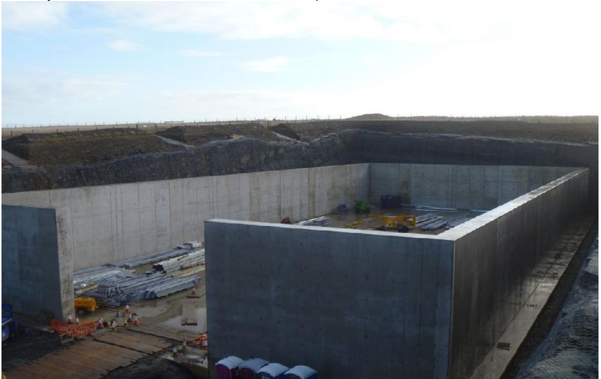
February 2013 – construction of re-inforced walls complete
