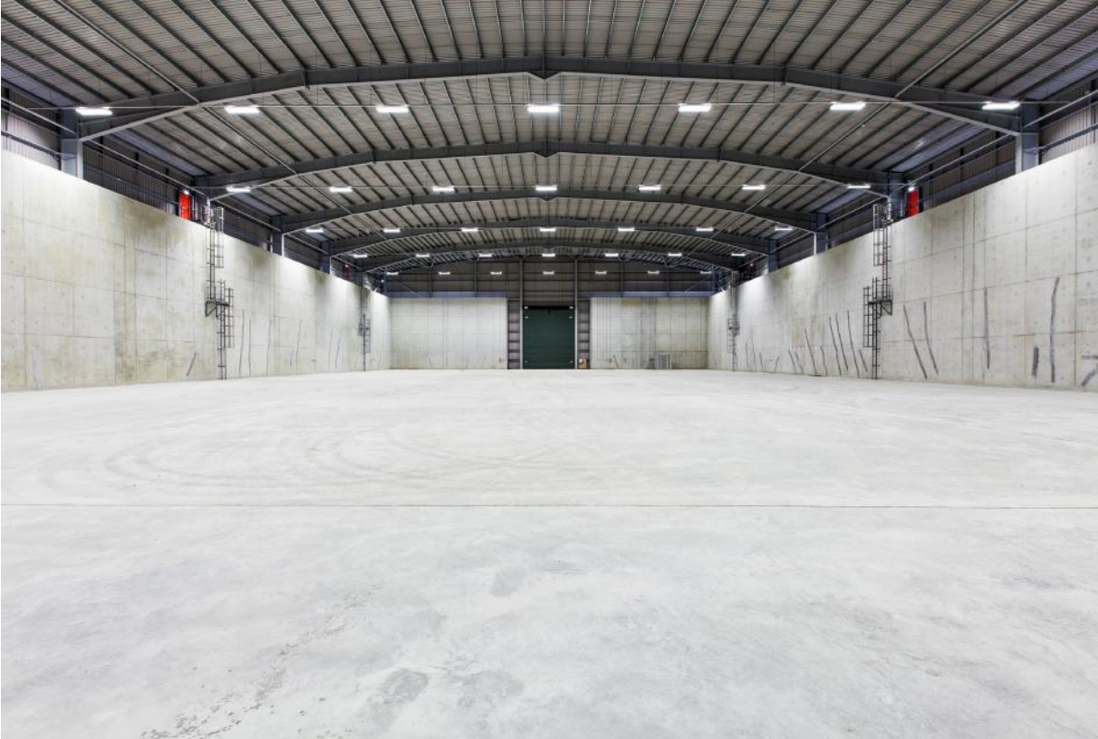
February 2014 – internal view of completed vault
