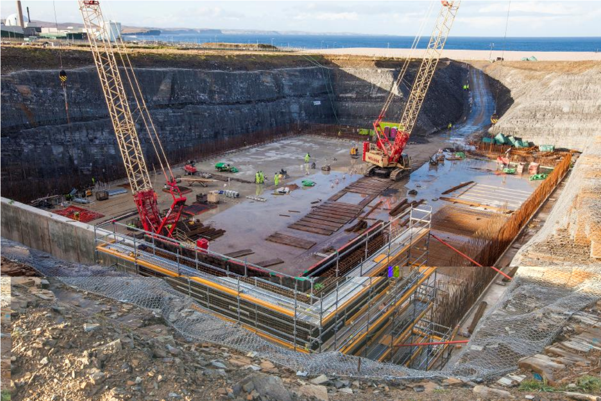
November 2012 – construction of re-inforced walls
