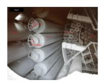
An off the shelf CCTV camera has provided crystal clear images of inside the reactor. Fifty years on from the construction of PFR, footage is being viewed that will allow the innards of the second (and last fast reactor) to be taken apart.
