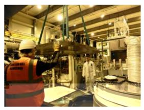
The PFR irradiated fuel cave (IFC) team installed a new adaptor plate. The new plate will facilitate the characterisation of waste packages as they are removed from the IFC. ILW shipments using the Z6016 flask have begun.
