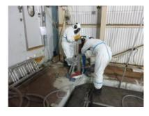
The bulk removal of NaK was completed in 2012 and, since then, work to remove the last of the coolant from the pipework and base of the structure has been undertaken. This final stage was extremely challenging because of the accessibility of the hazardous material.
