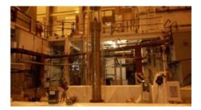
) The first of three water vapour nitrogen tools has been successfully installed and sealed into the reactor primary pump valve 2 penetration. Trialling of the next 2 in-reactor tools has commenced. The first of these is the rotor bucket grab tool which will remove the fuel tranfer rotor buckets (FTRB) from the reactor. The FTRGs are about 4 metrs in
